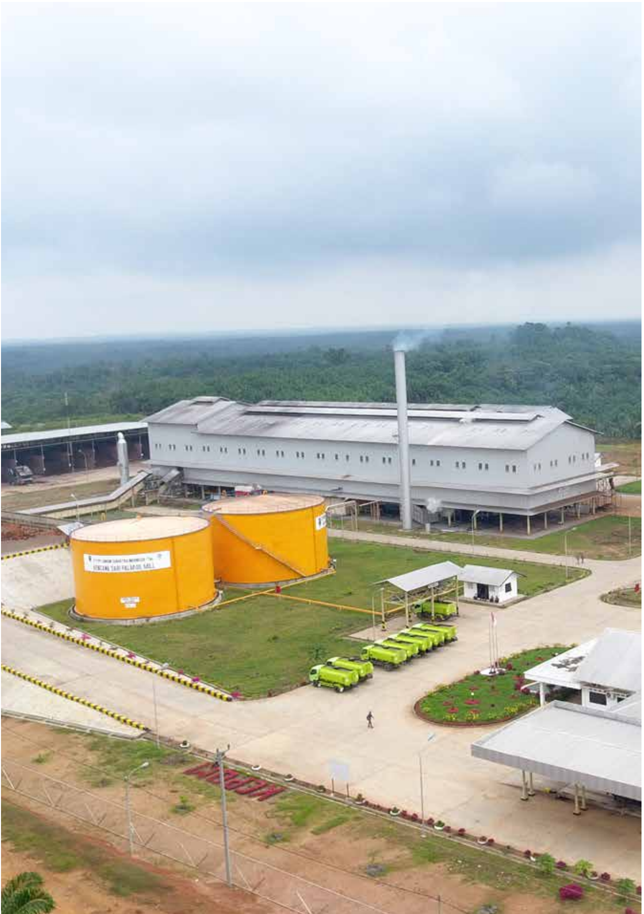
New Palm Oil Mill at South Sumatra Pabrik Kelapa Sawit Baru di Sumatera Selatan
