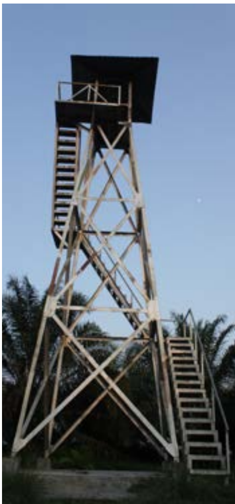
Fire Monitoring Tower at Turangie Estate, North Sumatra Menara Pengawas Kebakaran di Perkebunan Turangie, Sumatera Utara
