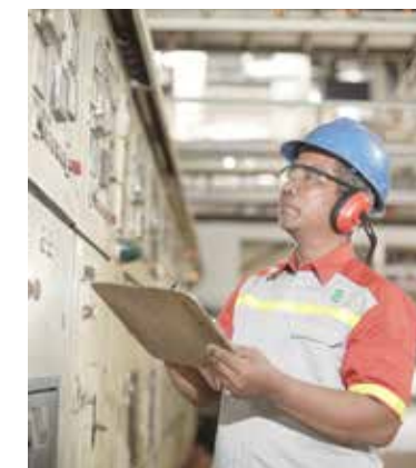
Energy consumption monitoring in our Begerpang Mill, Deliserdang, North Sumatra.
